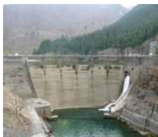
River maintenance flow discharge (Itoshiro Dam, Fukui Prefecture)
