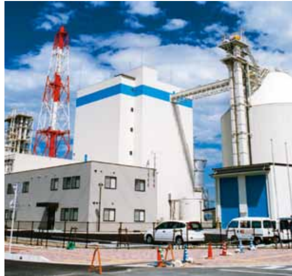
Omuta Recycle Power Station (Fukuoka Prefecture)
