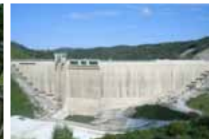
Dam built with “J-POWDER” (fly ash 3 ) as concrete admixture
