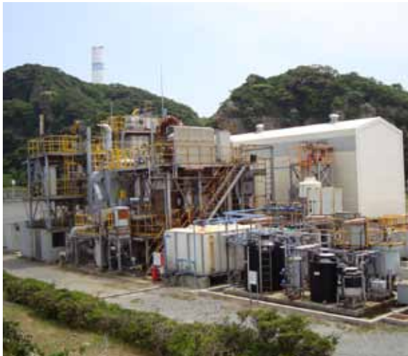
Test facilities for production of carbonized fuel from non-industrial waste (Matsushima Thermal Power Station, Nagasaki Prefecture)
