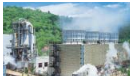
Onikobe Geothermal Power Station (Miyagi Prefecture)
