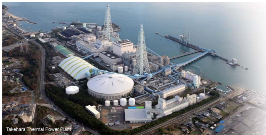
Takehara Thermal Power Plant
