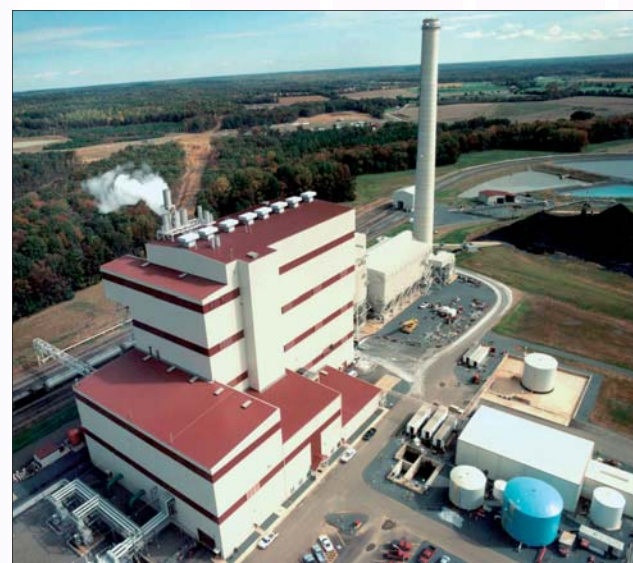
Birchwood Power Plant (USA)
