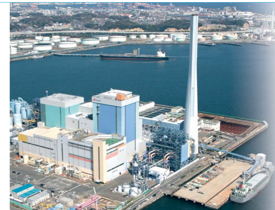
Isogo Thermal Power Plant
