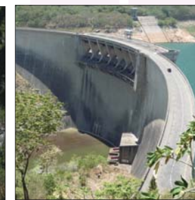
Victoria Hydropower Plant (Sri Lanka)
