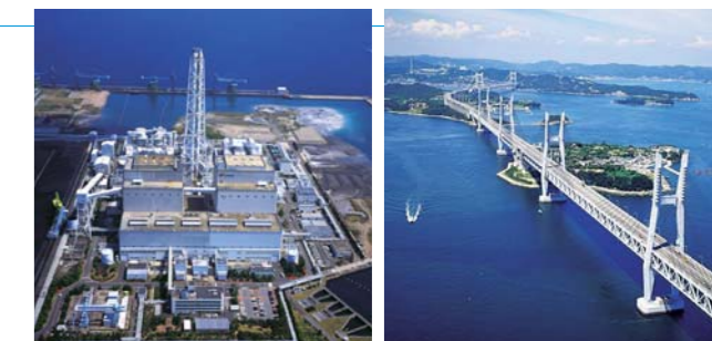
Matsuura Thermal Power Plant
