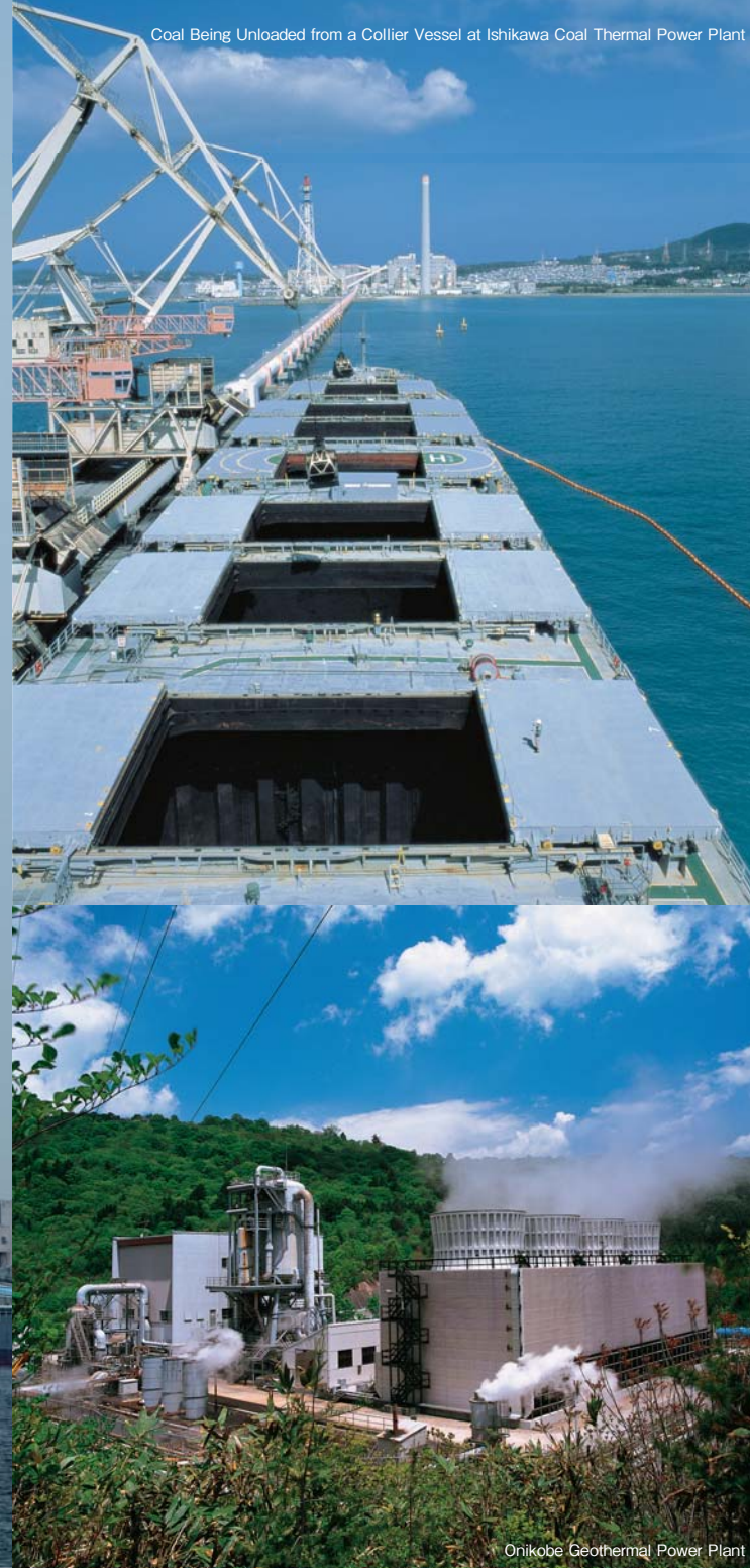
Isogo Thermal Power Plant
