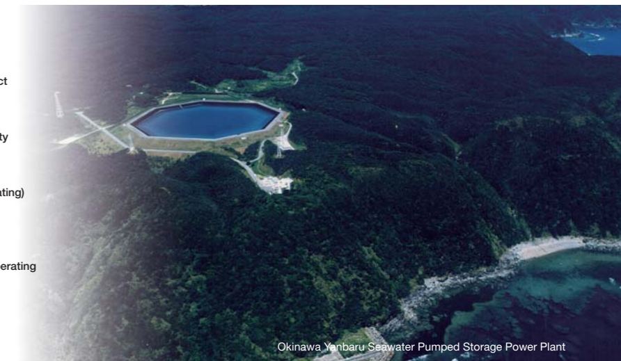
Okinawa Yanbaru Seawater Pumped Storage Power Plant
