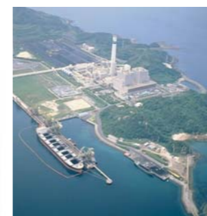
Matsushima Thermal Power Plant
