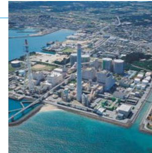
Ishikawa Coal Thermal Power Plant
