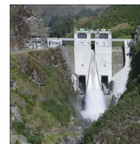
Yuncan Hydropower Plant (Peru)
