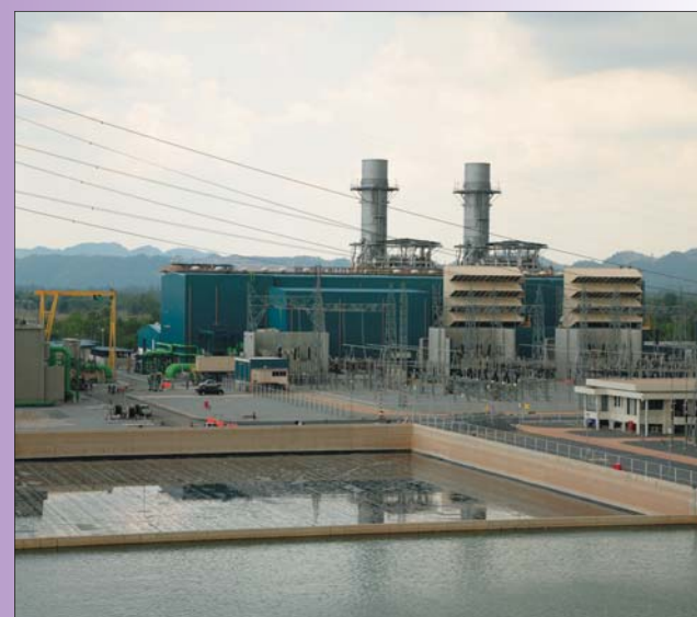
Kaeng Khoi No. 2 Gas-Fired Thermal Power Plant (Thailand)
