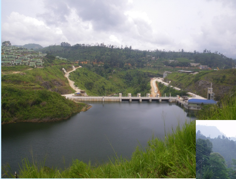
Talawakelle Intake Dam
