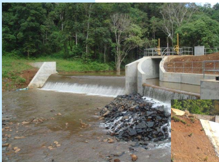
O'Romis Intake Dam
