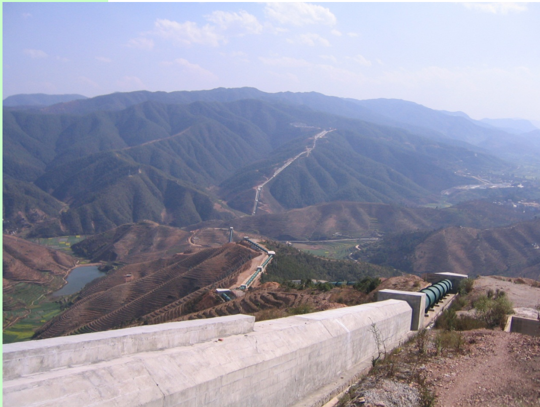
Water Supply Pipeline
