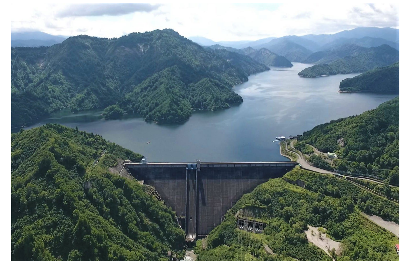
Okutadami, the largest capacity in Japan as a conventional hydroelectric power plant
