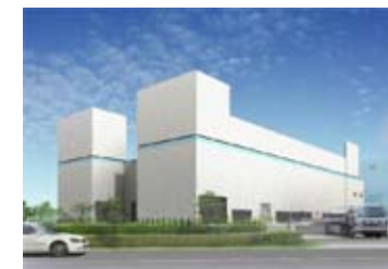
Facility for converting sludge into fuel (Hiroshima Pref.)
