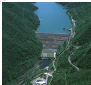
Miboro Power Plant (Gifu Pref.)
