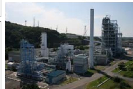
EAGLE Pilot Test Facility (Fukuoka Pref.)
