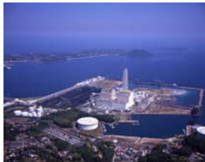
Matsuura Thermal Power plant (Nagasaki Pref.)
