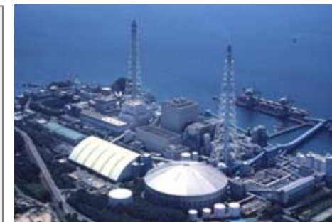
Takehara coal-fired Thermal Power Plant
