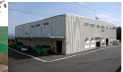
Wood biomass delivery Facility (Miyazaki Pref.)
