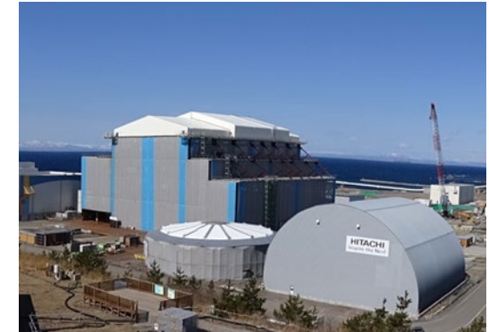
Status of construction (as of March 31, 2024)
