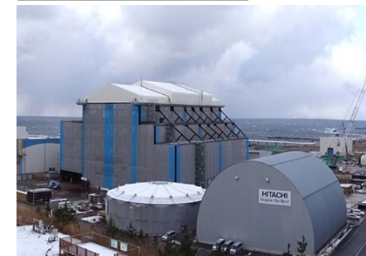
Status of construction (as of December 31, 2023)
