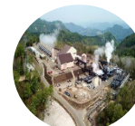
Wasabisawa Geothermal Power *3
