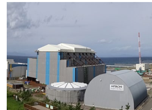
Status of construction (as of September 30, 2023)
