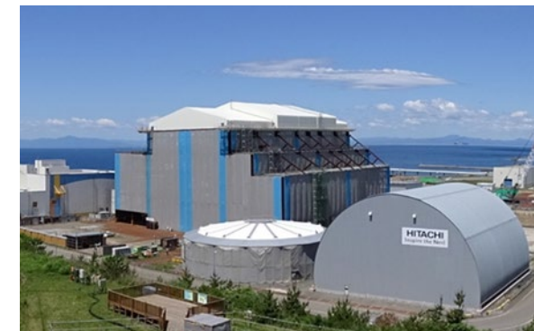
Status of construction (as of June 30, 2023)
