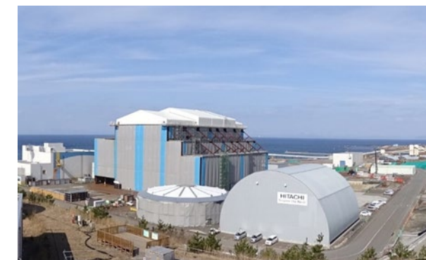
Status of construction (as of March ,31 2023)
