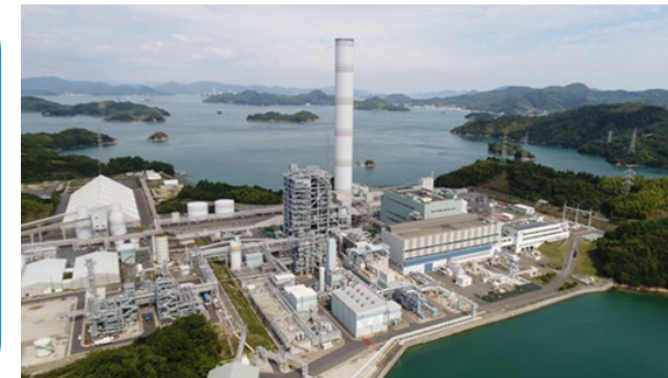
Fuel cell modules Solid Oxide Fuel Cell (SOFC) Capacity : 1.2MW class (0.6MW class SOFC X2)
