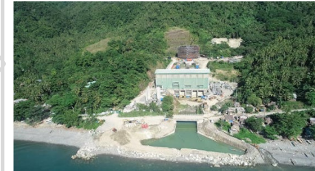
Lake Mainit Hydro (under construction)
