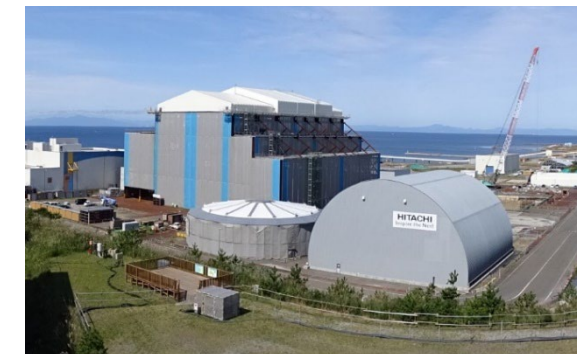
Status of construction (as of September 30, 2022)
