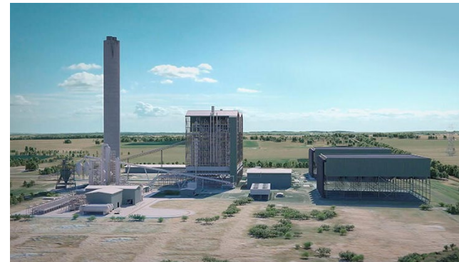
Rendered image of the proposed CO 2 capture plant and Millmerran Power Station in Queensland, Australia
