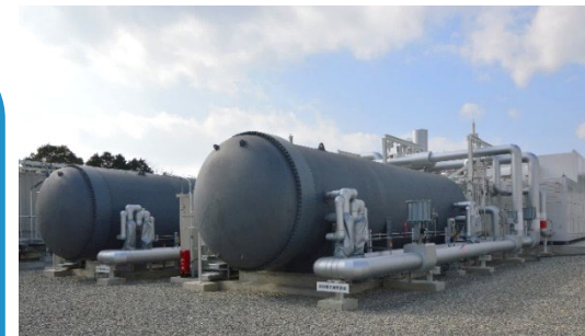
Fuel cell modules Solid Oxide Fuel Cell (SOFC) Capacity : 1.2MW class (600kW class SOFC X2)
