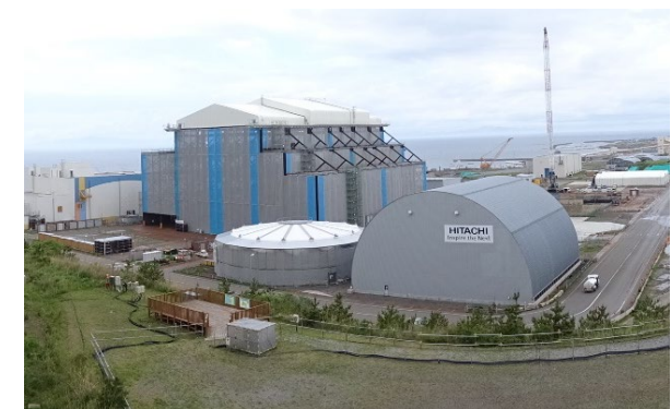
Status of construction (as of June 30, 2022)
