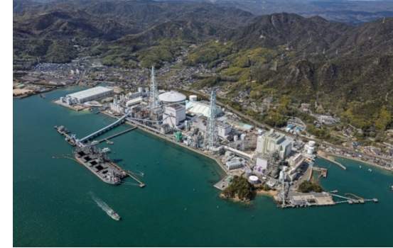
Takehara Thermal Power Plant New Unit No.1 and Unit No.3
