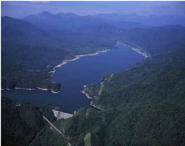
Nukabira Dam (Hokkaido prefecture)
