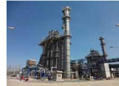
KP1 (Jan. 2013, in operation)
