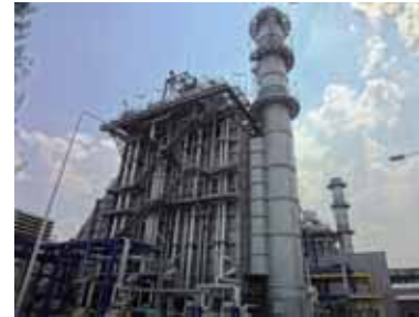
TLC (Mar. 2013, in operation)
