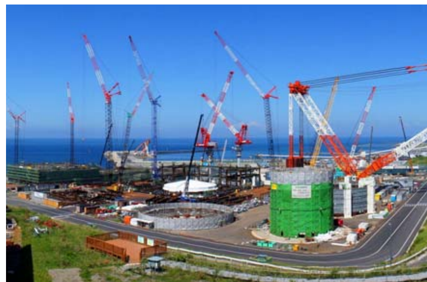
Construction site (as of September 2010)
