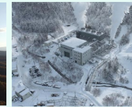
Miyagi-Onikobe Geothermal Power Plant Owned capacity: 14.9 MW
