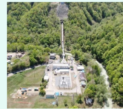
Hokkaido-Shinkatsurazawa Power Plant (Hydroelectric) Owned capacity: 16.8 MW
