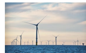
Triton Knoll Offshore Wind Farm (Commercial operation began in 2022)
