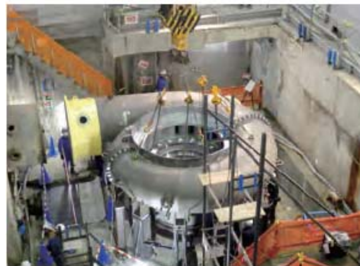
Installing a waterwheel casing for construction of Shin-Katsurazawa Power Station
