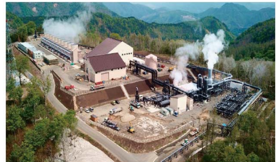
Wasabizawa Geothermal Power Plant commenced operation
