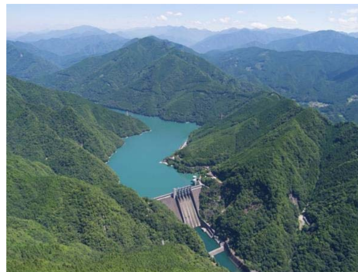
Sakuma Dam (Shizuoka)
