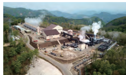
Wasabizawa Geothermal Power Plant (Akita Prefecture)
