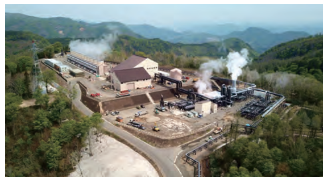
Wasabizawa Geothermal Power Plant (Akita Prefecture)
