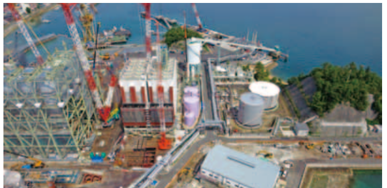
Under construction for replacement
