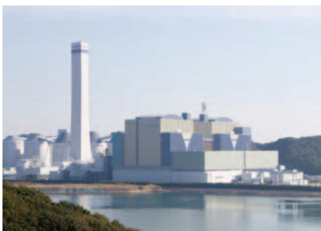
Tachibana Thermal Power Plant
