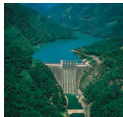
Sakuma Power Plant (Shizuoka Prefecture)
