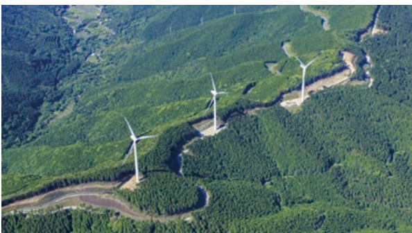
Minami Ehime Wind Farm
