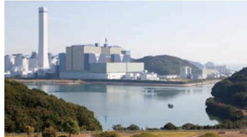
Tachibanawan Thermal Power Plant
