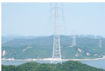
Honshu-Shikoku Interconnection (Okayama and Kagawa Prefectures) 500,000-volt transmission lines across the Seto Inland Sea to connect Honshu and Shikoku. These transmission lines are connected to backbone transmission lines in Honshu and Shikoku, contributing to stable electric supplies in western Japan.
