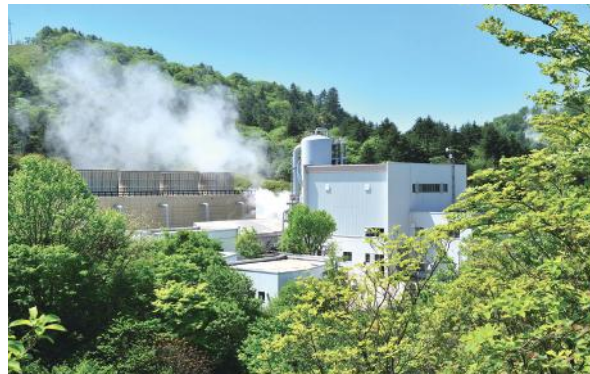
Onikobe Geothermal Power Station (Miyagi Prefecture)
