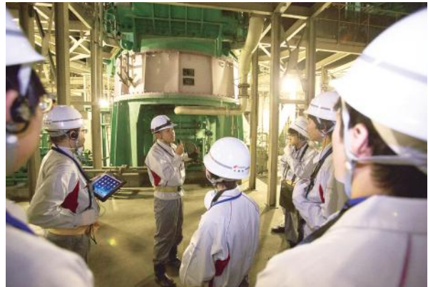
Participants hear explanations from employees who actually work in the power plant
