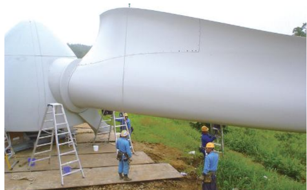
Assembling a wind turbine (the vane portion)
