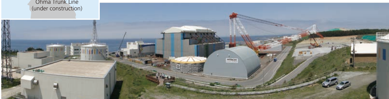
Construction status of the Ohma Nuclear Power Project (photographed in July 2015)
