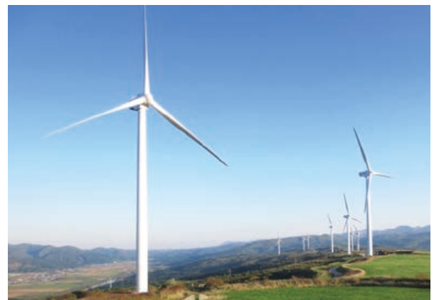
Kaminokuni Wind Farm (Hokkaido Prefecture)
