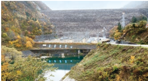
Miboro Power Plant (Gifu Prefecture)
