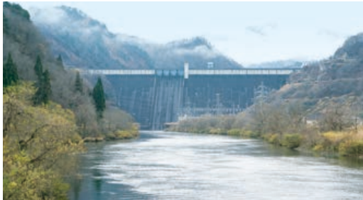
Tagokura Power Plant (Fukushima Prefecture)
