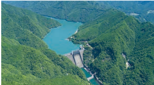
Sakuma Power Plant (Shizuoka Prefecture)
