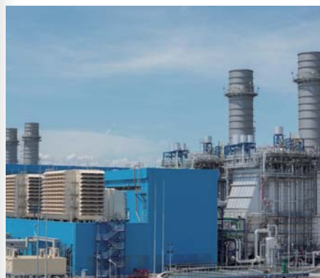
Nong Saeng Power Project Unit No. 1 Power Plant (Thailand)
