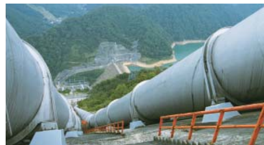
Okukiyotsu Power Plants (Niigata Prefecture)
