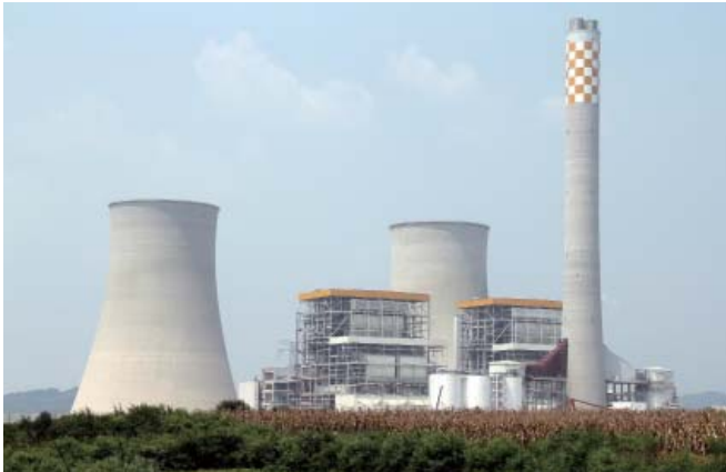
Hezhou Power Plant (China)
