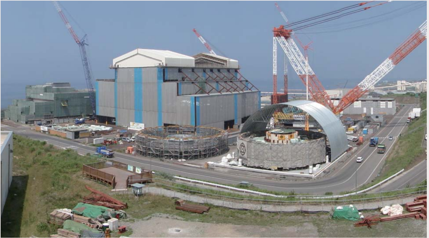
Construction status of the Ohma Power Project (photographed in July 2014)
