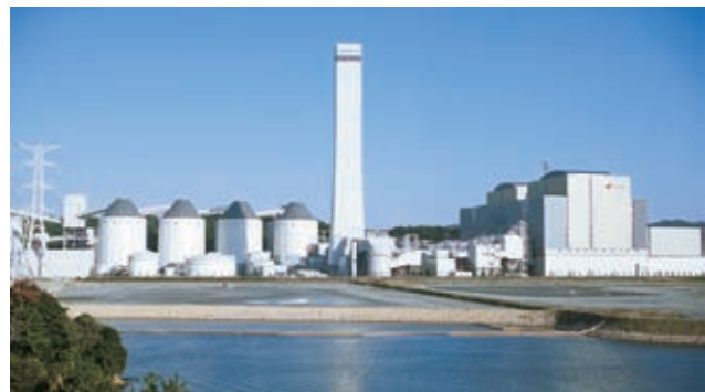
Tachibanawan Thermal Power Plant (Capacity 2,100 MW, Tokushima Prefecture)
