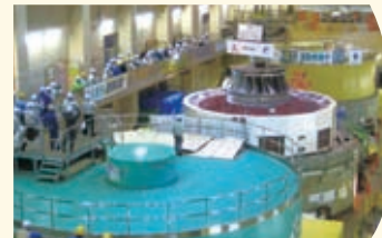
Upgrade of Tagokura Power Plant No. 3
