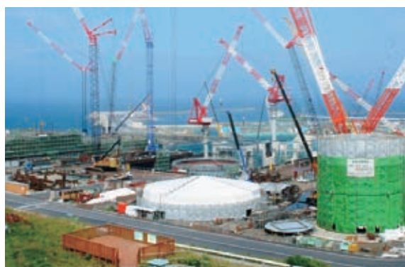
Construction work (as of July 2010)
