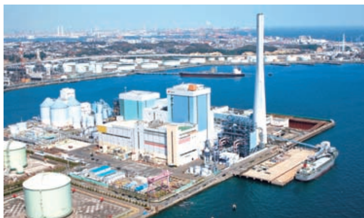
Isogo Thermal Power Plant (after replacement)
