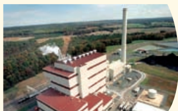
Birchwood Coal-Fired Thermal Power Plant
