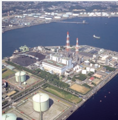
Isogo Thermal Power Plant: operations launched in 1967
