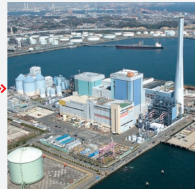
New No. 1 Plant: operations launched in 2002 New No. 2 Plant: operations launched in July 2009
