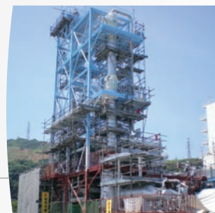
CO 2 separation and recovery facility (under construction)
