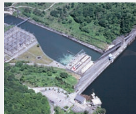
Tagokura Power Plant (Fukushima Prefecture)
