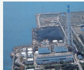
Takasago Thermal Power Plant (Hyogo Prefecture)
