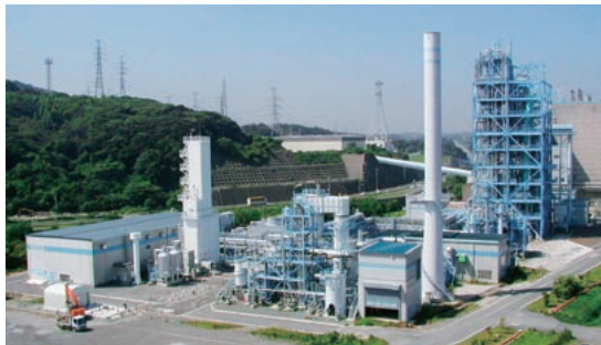
EAGLE pilot-scale testing facilities (Wakamatsu Research Institute, Fukuoka Prefecture)
