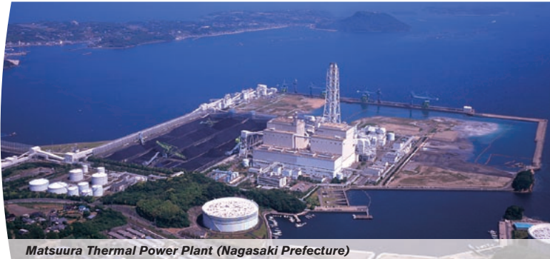
Matsuura Thermal Power Plant (Nagasaki Prefecture)
