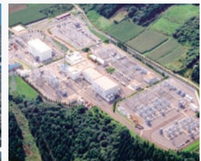
Kitahon Linkage Facilities and Hakodate AC/DC Converter Station (Hokkaido)
