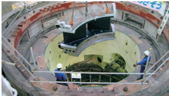
Comprehensive upgrade of main machinery and equipment at Tagokura Power Plant
