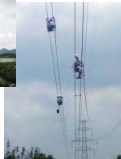
Inspecting the Kumano Main Transmission Line in Nara Prefecture
