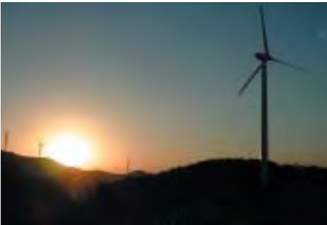
Nagasaki-Shikamachi Wind Farm (Nagasaki Prefecture)
