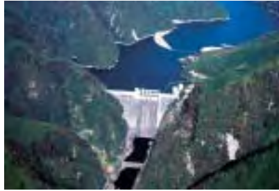
Sakuma Power Station (Shizuoka Prefecture)
