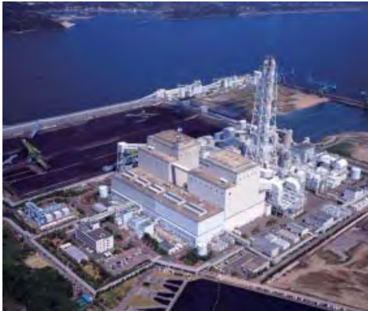
Mitsuura Thermal Power Station (Nagasaki Prefecture)
