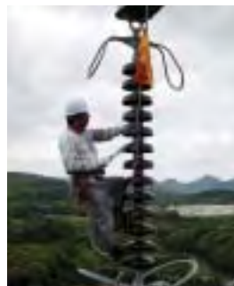
Inspection of insulators on the Matsushima Thermal Line in Nagasaki Prefecture
