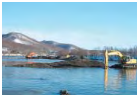
Sediment dredging at Senbiri Dam (Hokkaido Prefecture)
