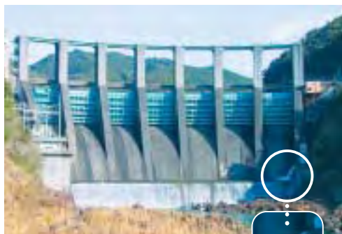
River maintenance discharge (circled area) at Nanairo Dam (Wakayama Prefecture/Mie Prefecture)
