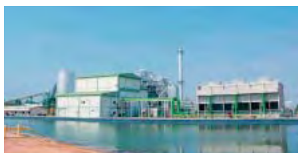
Roi-Et Rice-Chaff-Fired Thermal Power Generation Plant (Thailand)
