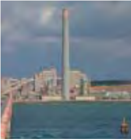
Ishikawa Coal-fired Power Station (Okinawa Prefecture)
