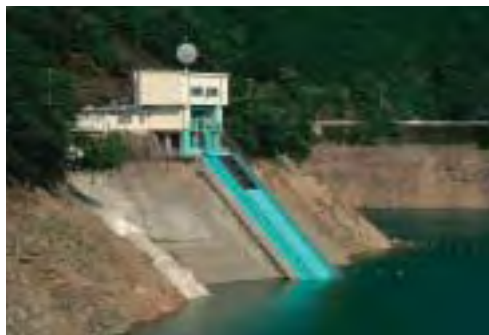
Sakamoto Dam surface-water intake system under construction (Nara Prefecture)
