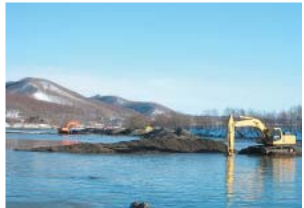
Sediment dredging at Senbiri Dam (Hokkaido Prefecture)
