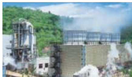
Onikobe Geothermal Power Station (Miyagi Prefecture)
