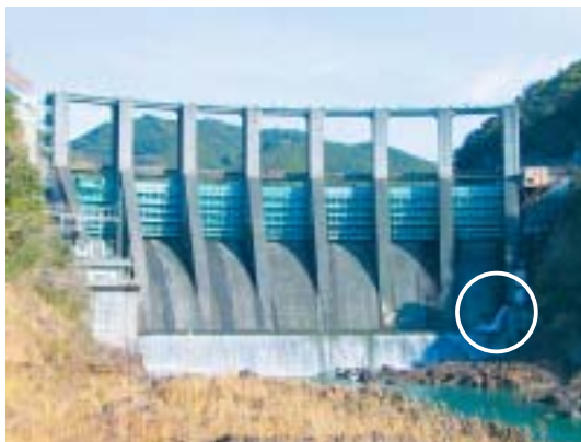
Maintenance flow discharge (circled area) at Nanairo Dam (Wakayama Prefecture/Mie Prefecture)
