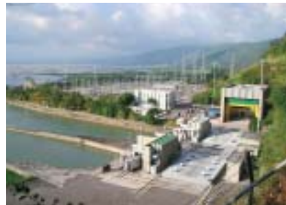
Calayan Pumped-water Power Generation Plant (Philippines)
