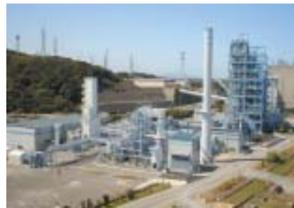
Pilot plant testing technology to produce coal gas suitable for fuel cells (Fukuoka Prefecture)
