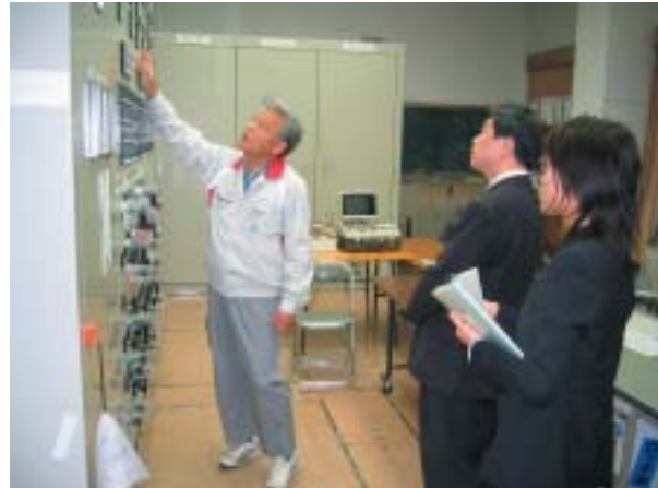
On-site review (Nukabira Power Station, Kamishihoro Power Administration Office)
