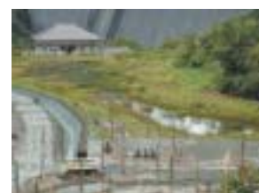
Wetland restoration following completion of Okutadami-Otori hydro project construction
