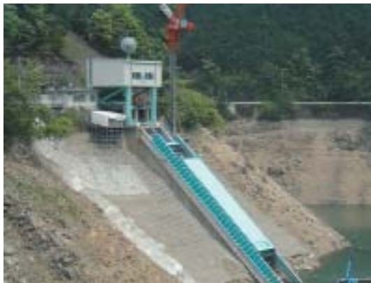
Sakamoto Dam surface-water intake system under construction (Nara Prefecture)
