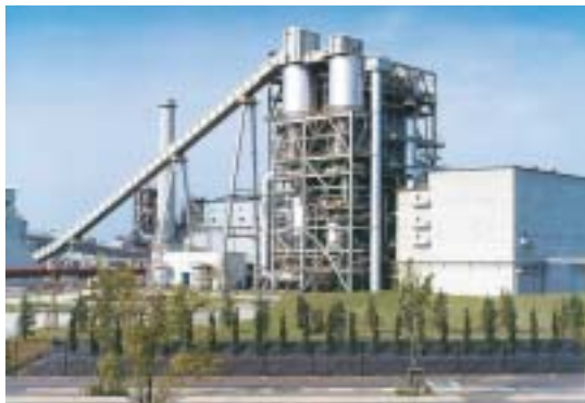
Itoigawa Power Station (Niigata Prefecture)
