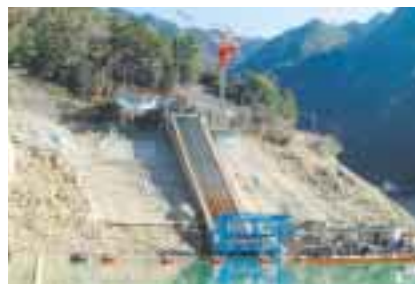
Sakamoto Dam's surface intake facilities under construction (Nara Prefecture)
