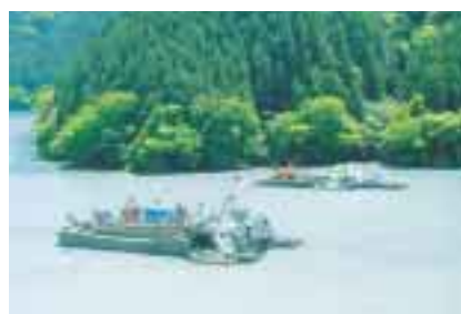
Removal of sedimentation in the Akiba Dam (Shizuoka Prefecture)
