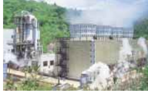
Onikobe Geothermal Power Station (Miyagi Prefecture)
