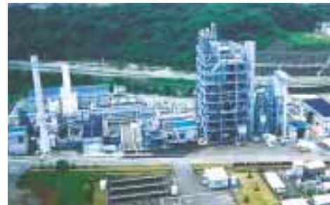
Coal Energy Application for Gas, Liquid & Electricity pilot plant
