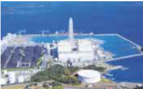
Matsuura Thermal Power Station (Nagasaki Prefecture)
