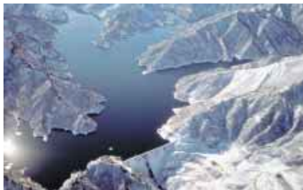
Okutadami Power Station (Fukushima and Niigata)
