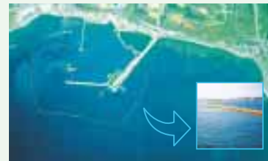
Protective barrier to prevent the spread of pollution
