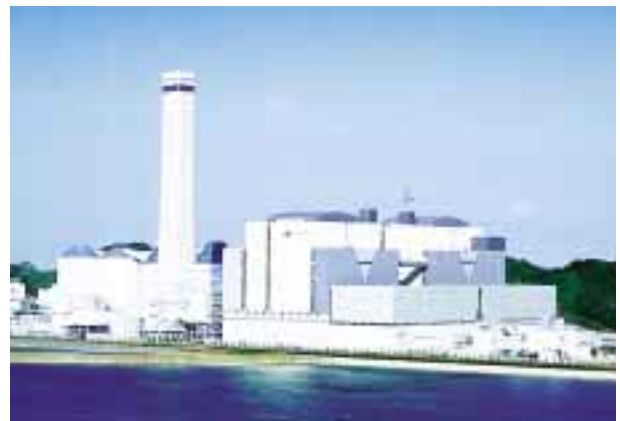
Tachibana Wan Thermal Power Station (Tokushima Prefecture)
