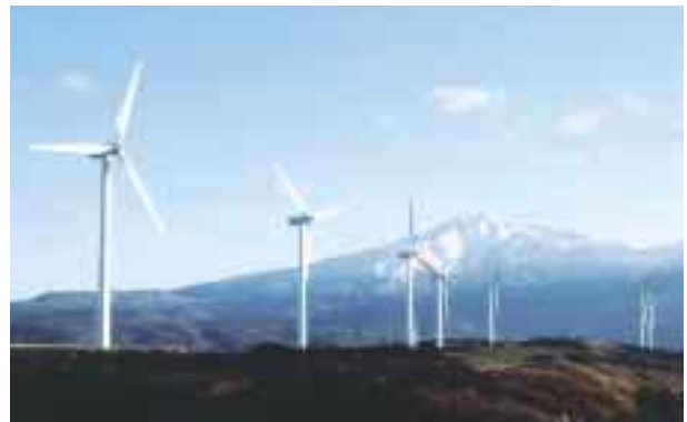
Nikaho Kogen Wind Farm (Akita)
