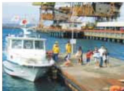
Matsushima Thermal Power Station, (Nagasaki Prefecture)
