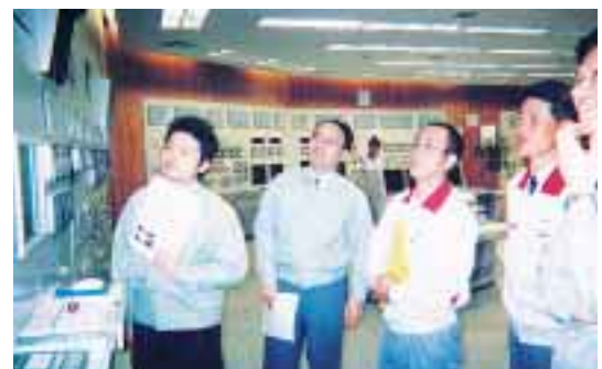
Matsuura Thermal Power Station (central control room)
