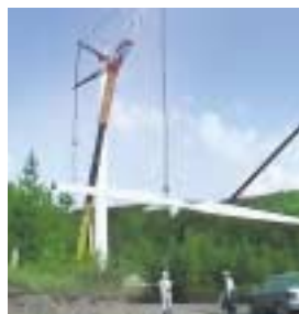
Installing a turbine blade at Green Power Kuzumaki Wind Power Station.
