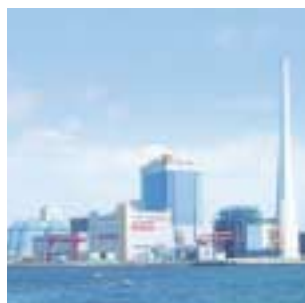
In April 2002, we completed replacement work and began operations at the No. 1 unit of the Isogo Thermal Power Station. We plan to construct the No. 2 unit, which is scheduled to go on line in July 2009.
