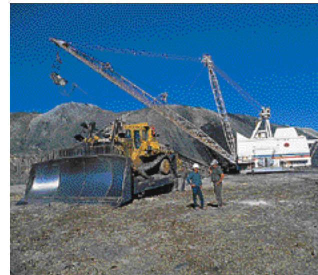
Blair Athol Coal Mining Project in Australia
