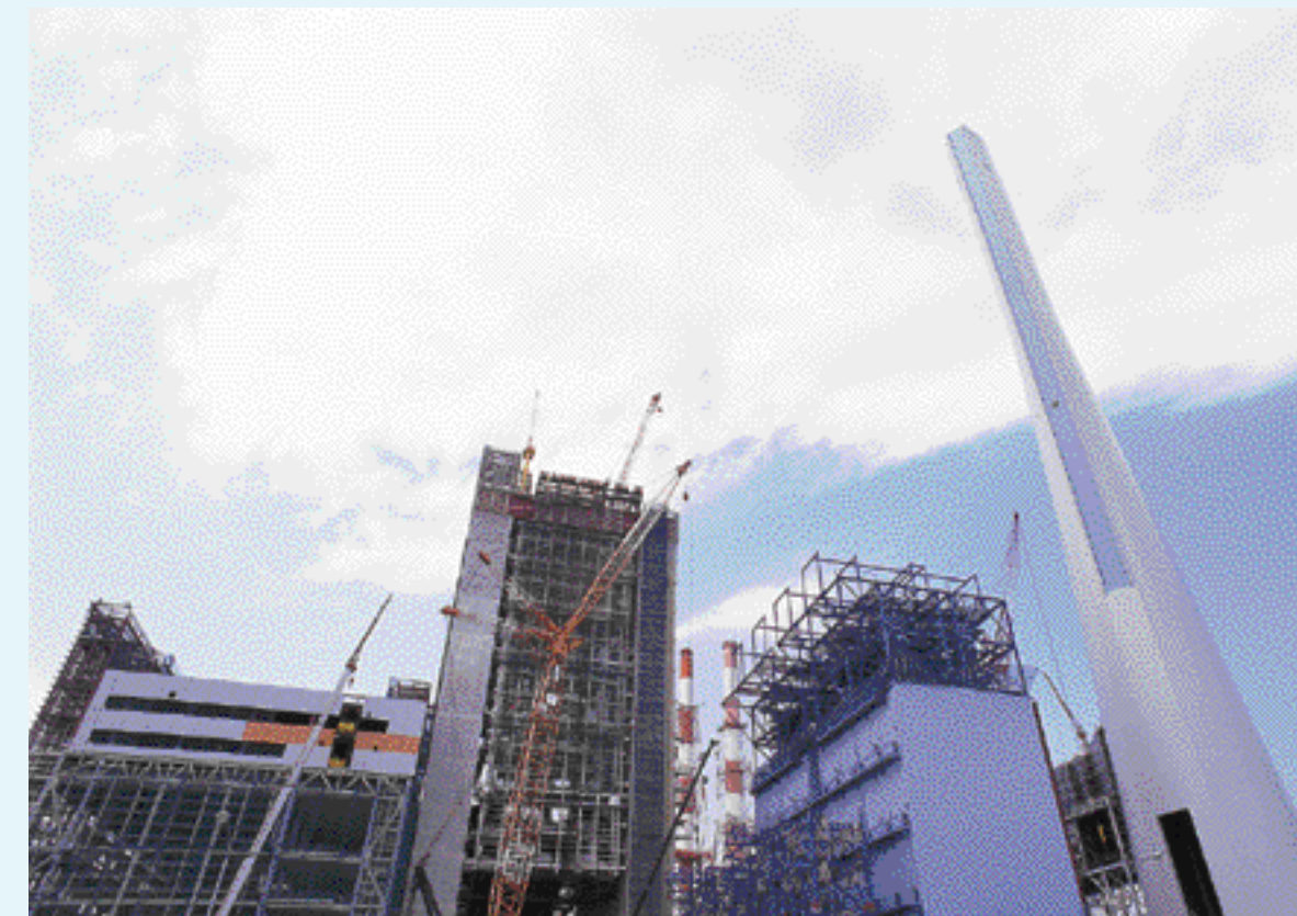
Isogo Thermal Power Station ( Under Construction for Replacement )
