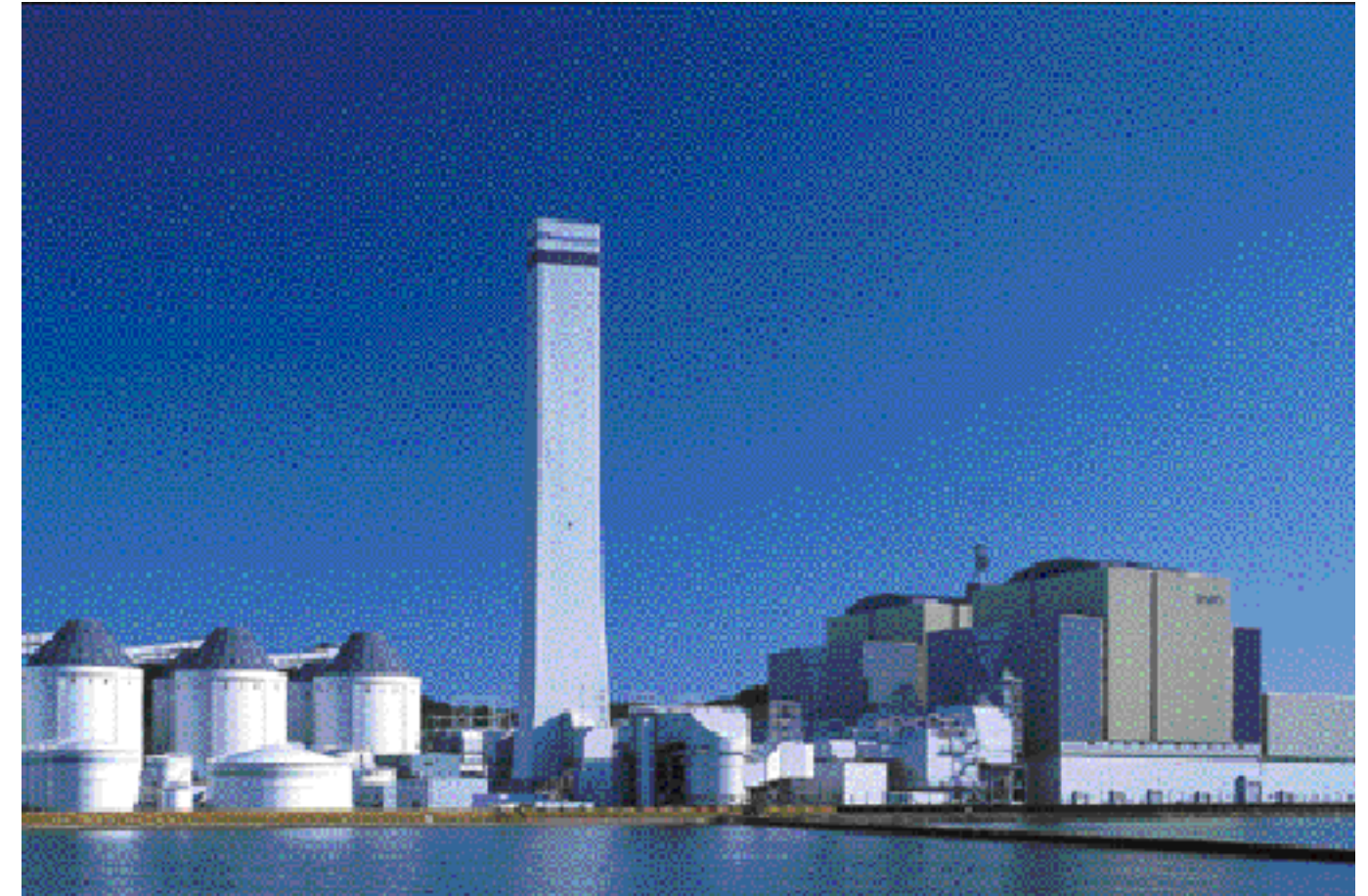
Tachibanawan Thermal Power Station, Tokushima Prefecture
