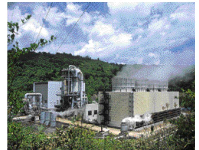
Onikobe Geothermal Power Station, Miyagi Prefecture
