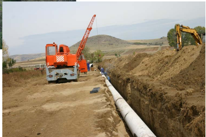
Water Supply Pipeline
