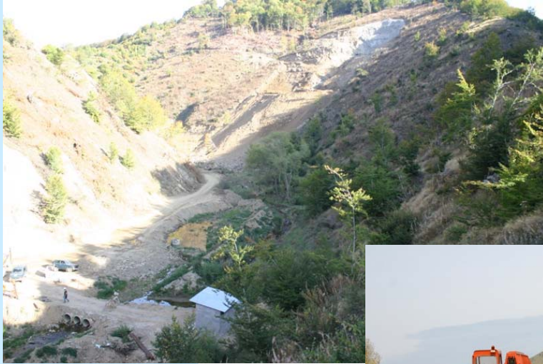
KNEZEVO Dam Site
