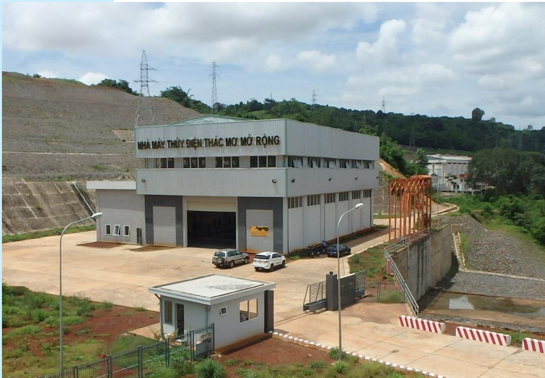
New Powerhouse in the foreground and Existing Powerhouse in the background
