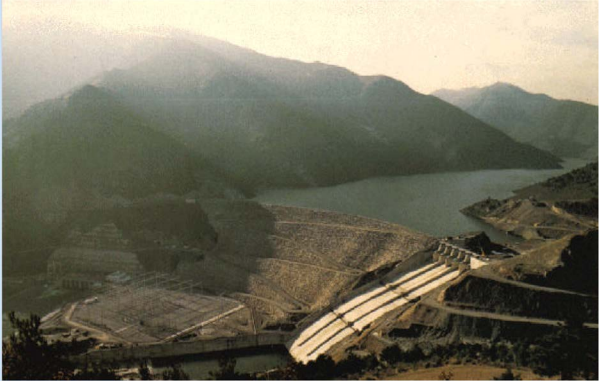
General View of Altinkaya Project
